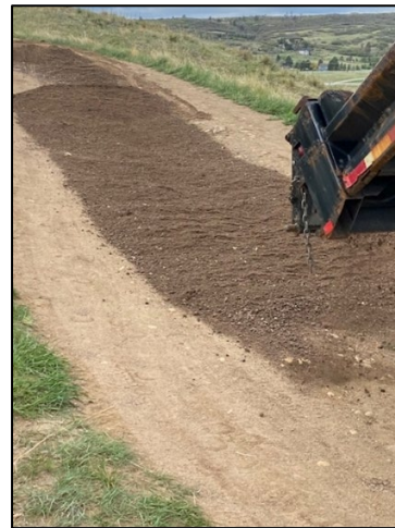
Grading and compacting for trail repair
