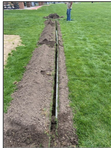
Staff rerouting irrigation lines
