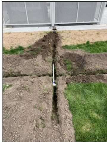
Reconfiguring irrigation next to the restroom structure
