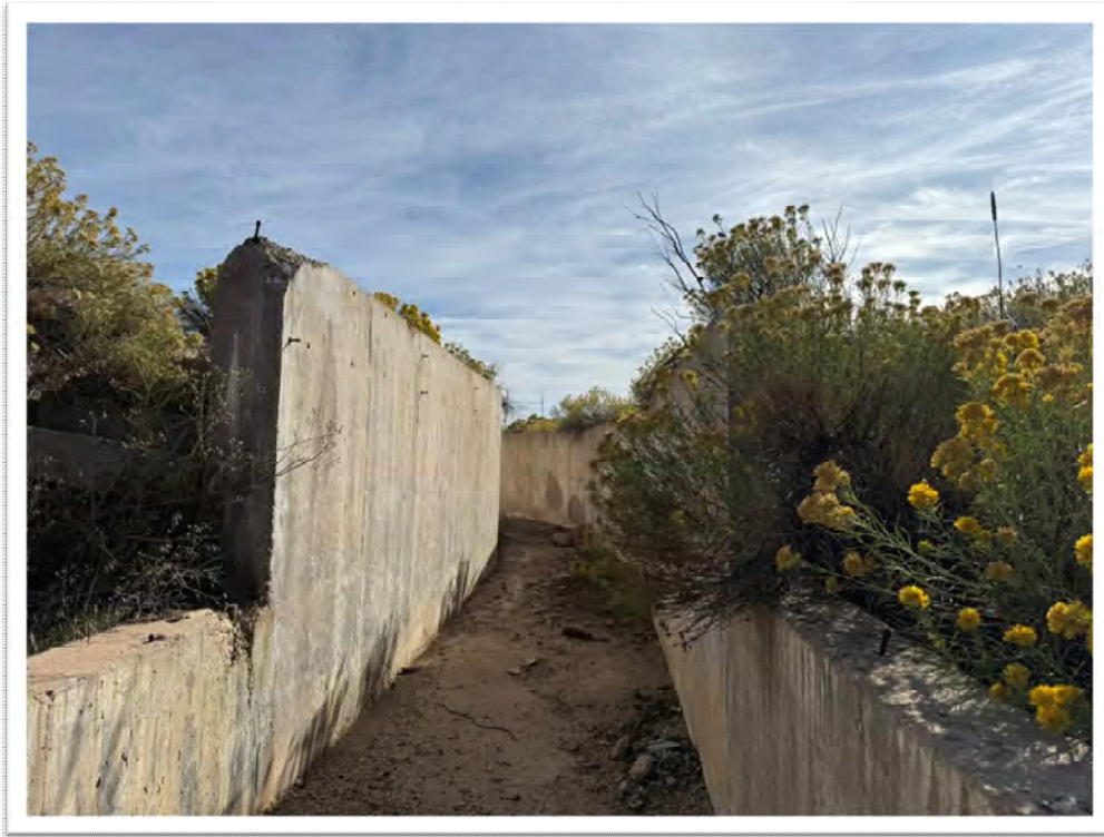
Concrete walls adjacent to the eastern boundary (offsite).
