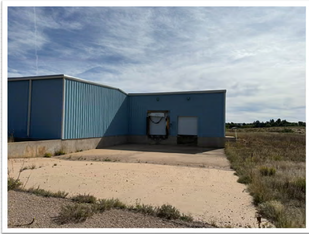
Blue maintenance shed (offsite).
